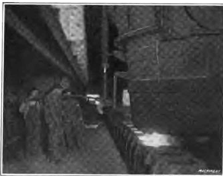
Fig. 5. Casting Crew on Open-hearth Pouring Platform filling Molds with Molten Steel tapped through Bottom of Ladle
